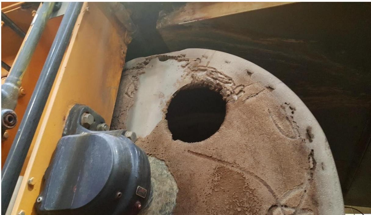
*Image 1 – Struvite Removed in Areas Prior to HydroFLOW Installation*
