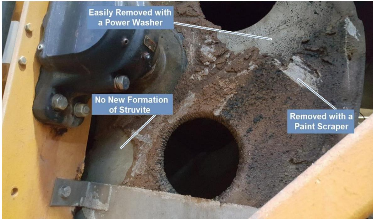
**Image 3** – *HydroFLOW has Prevented New Struvite and Caused Easy Removal of Existing Struvite*
